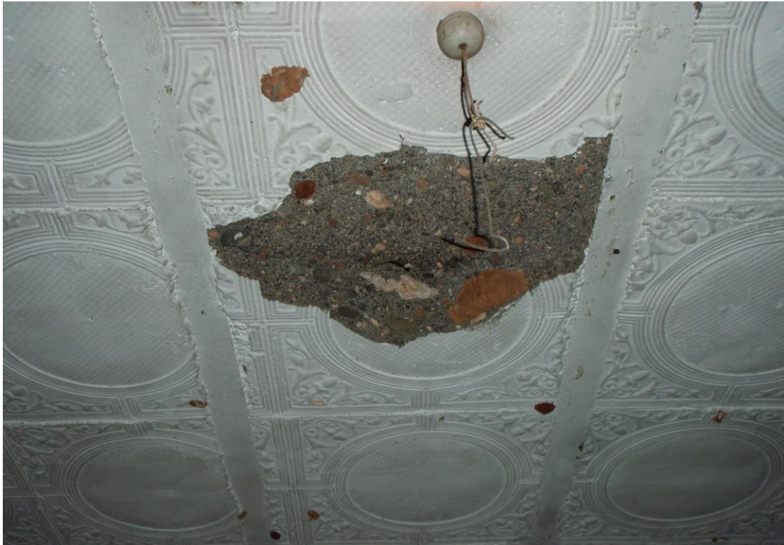
Concrete roof with pressed tin design, 2012
