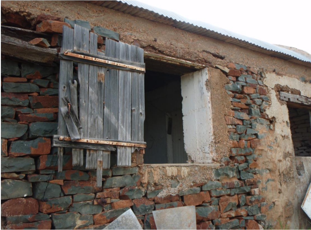
Kitchen and mess for workers, 2012
