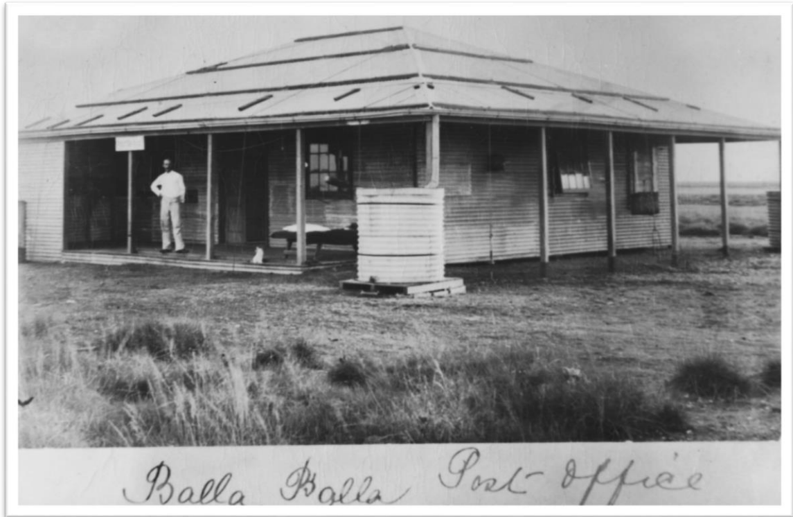
Image 8. Balla Balla Post Office 1898, note the steel cyclone tie-downs (Courtesy Shire of Roebourne Local History Collection, 2005.120)
