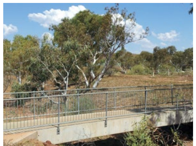
Image 76. Existing drainage swale in Pegs Creek
