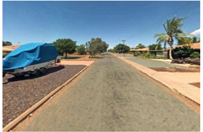
Image 29. Existing View of Streetscape
